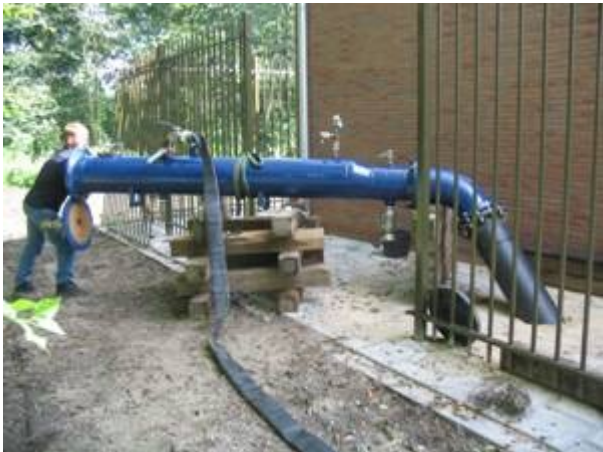
Launching area at the pump station.
