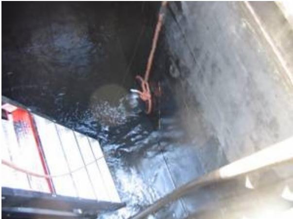
Retrieval of the inspection pig in the Septic tank
