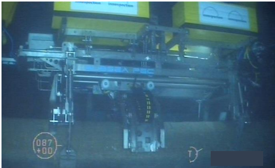
Figure 10: Subsea Pulsed Eddy Current equipment deployed on subsea pipeline
