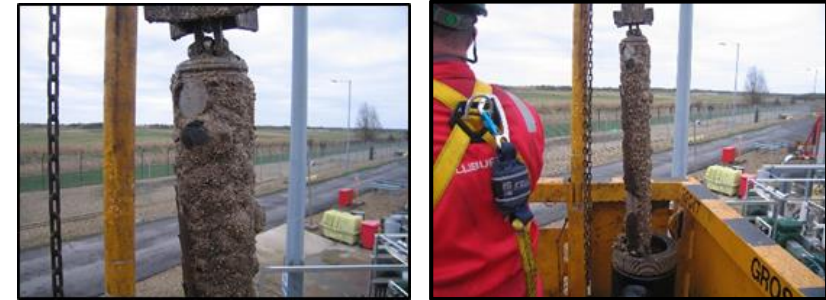
Debris Removed from 4" MeOH 118.7km Pipeline
