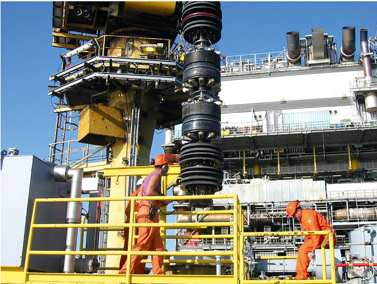
Figure 15. 30 inch SmartPlug ready to enter the vertical pig launcher
