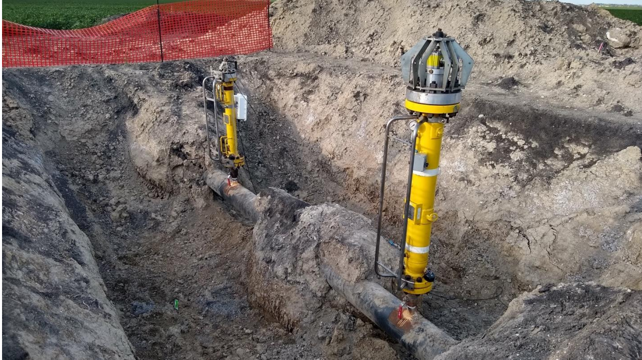
Figure 5: In-line Charging Site on 10 inch Pipeline
